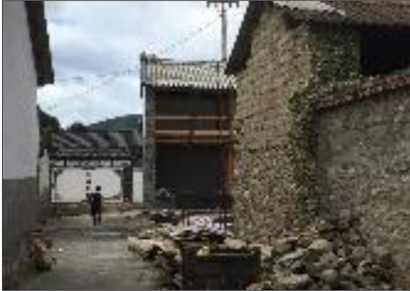
Figure 1: New house being constructed next to an old stone one.
